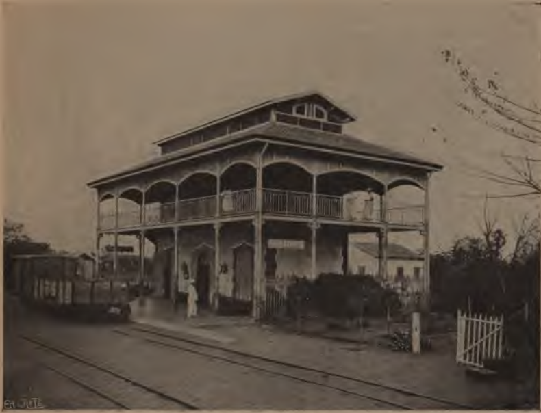
STATION DE PIHE-GOUREVE.
