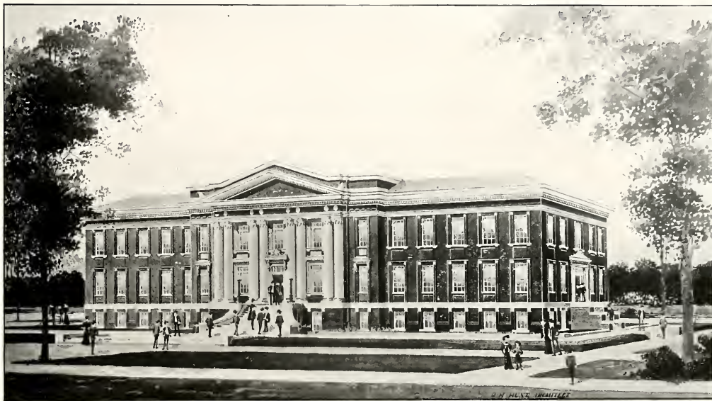
NEW BUILDING NOW UNDER CONSTRUCTION WILL BE READY FOR NEXT TERM
