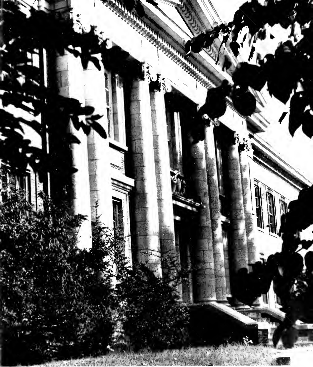
The Administration Building
