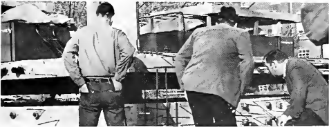
It was a little over a year ago that Blythe Hall looked like this. Inch by inch, the building was lifted hydraulically off the ground.
