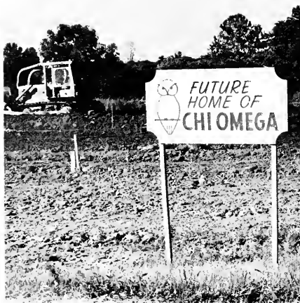
Construction begins on Chi Omega house.
