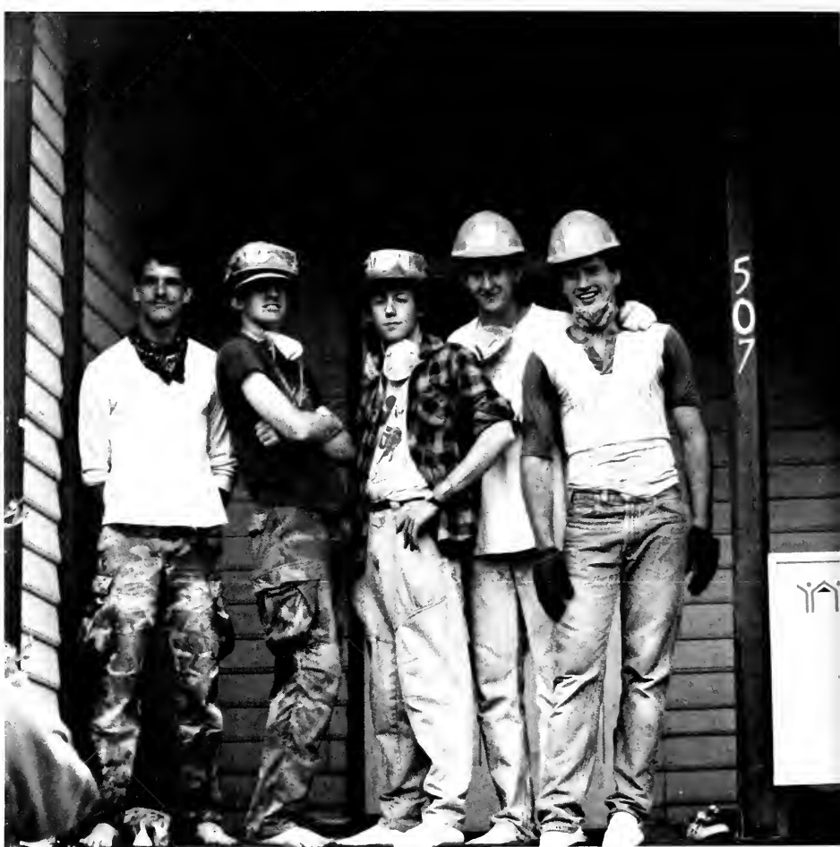
Doug Sander, Ken Wiandt, David Duncan, "Bif" Dickerson, and Tim Canfield show-off their attire after demolishing a house for Habitat for Humanity during their spring break as a part of S.P.O.T.S.
