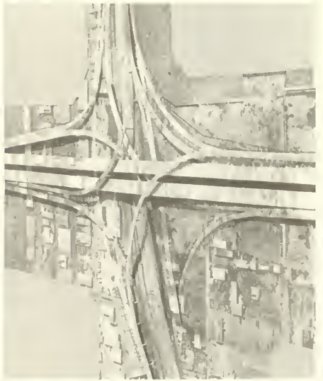
I-10/I-17 Interchange, Phoenix, AZ.
