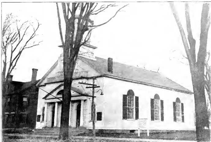
UNITARIAN CHURCH, SACO which John Fairfield was instrumental in founding and which the Fairfield family attended
