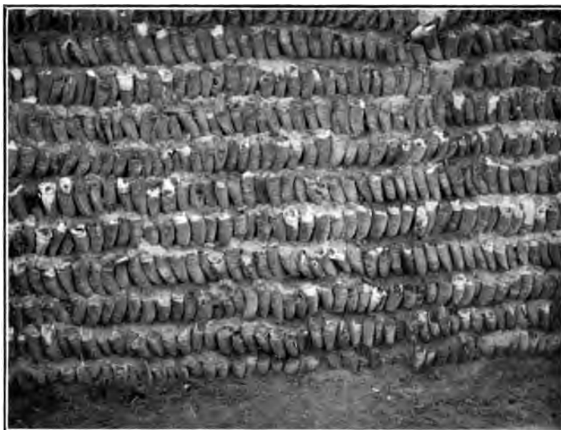
This is an example—the best in Lhasa—of the famous horn-masonry which is characteristic of the place, and noted by every traveller to the city.
