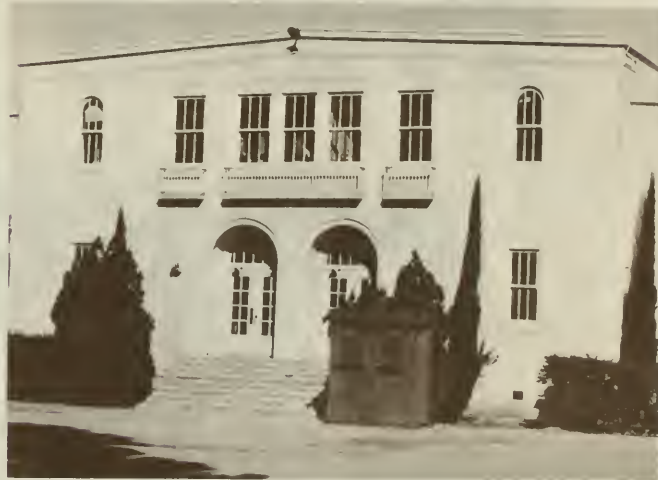
THIS fine old building had to be bull-dozed in the late 60's because of a state law-Field At. It served as a second gym and locker room.
