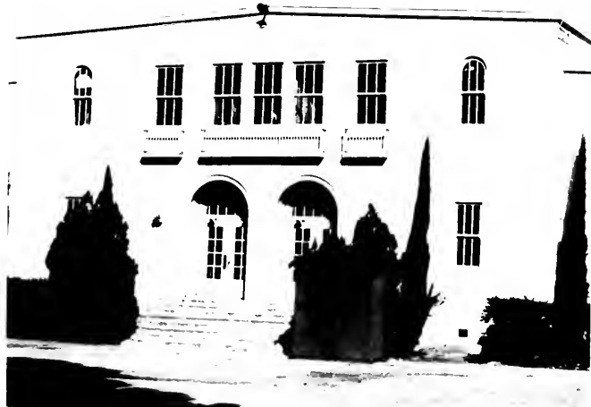
THIS fine old building had to be bull-dozed in the late 60's because of a state law-Field At. It served as a second gym and locker room.
