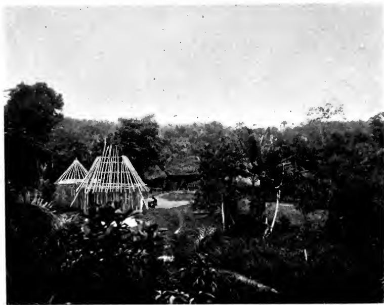
387. VAI HOUSES IN PROCESS OF CONSTRUCTION
