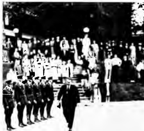
1939: DEDICATION OF THE ARTS BUILDING. Gov. Earle is in the foreground.
