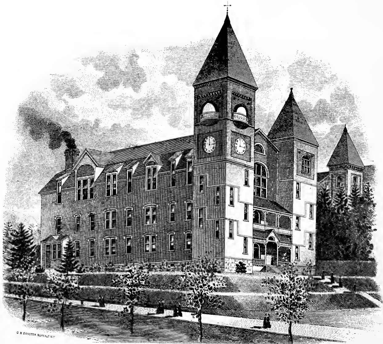
Construction of Alumni Hall
