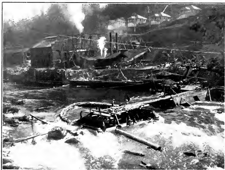
CONSTRUCTING DAM ABOVE SNOQUALMIE FALLS.
