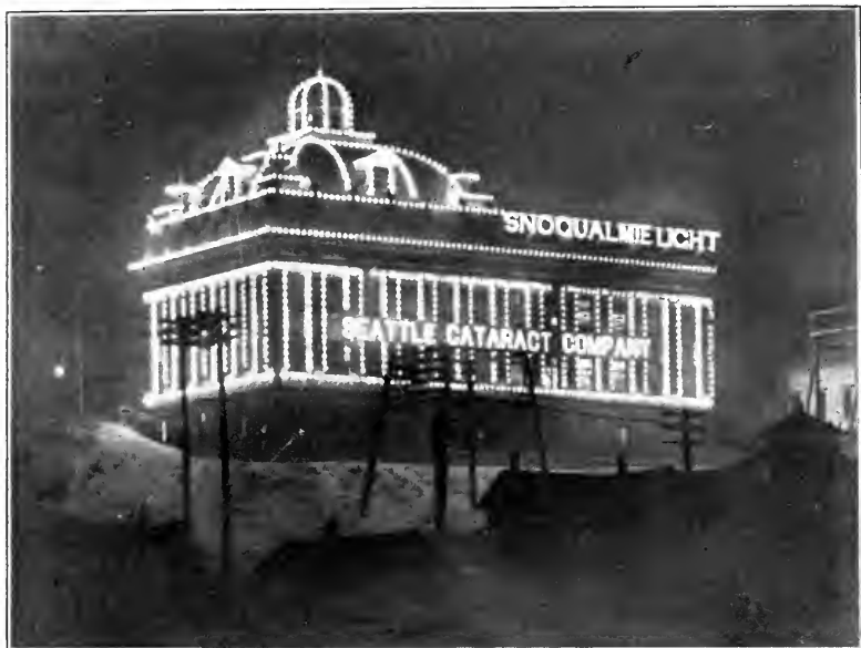
SEATTLE SUBSTATION AND GENERAL OFFICES.
