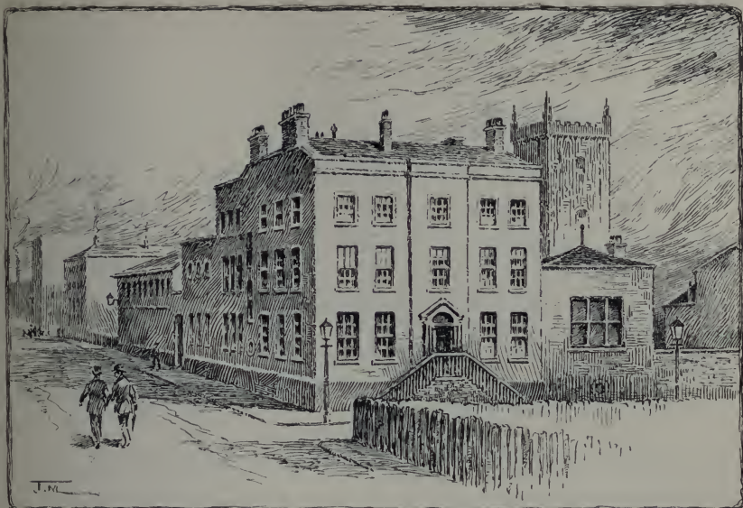
THE OLD OWENS COLLEGE, QUAY STREET, MANCHESTER.
