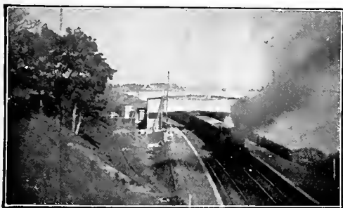
ELEVATED CROSSING FOR PASSENGERS.
