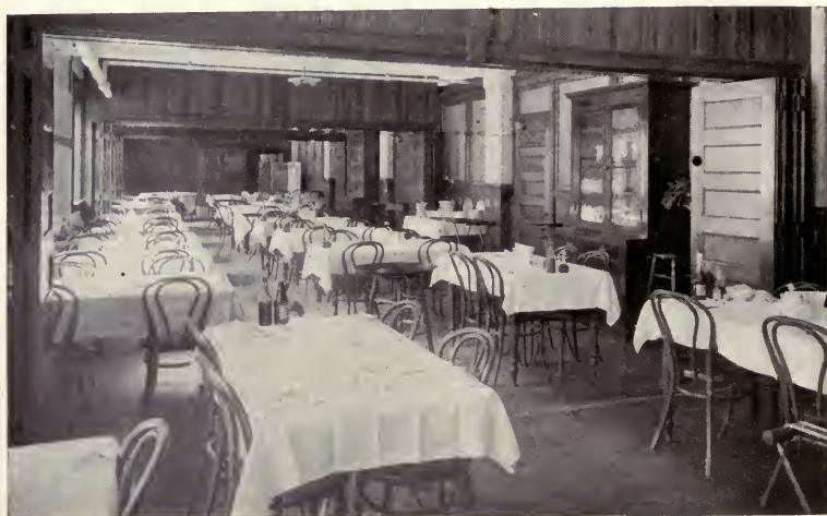
Fig. 59. DINING ROOM, MAIN OFFICE BUILDING, SCHENECTADY WORKS
