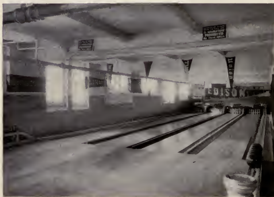
Fig. 6. BOWLING ALLEYS OF THE EDISON CLUB WITH THEIR AUTOMATIC PIN-SETTING EQUIPMENT. INTERCOLLEGIATE BOWLING TEAMS HAVE ROUSING TIMES IN THEIR MATCHES
