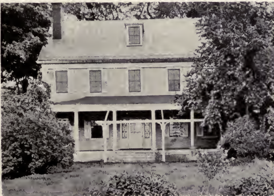
Fig. 16. IT IS A HANDSOME BUILDING, FORMERLY THE RESIDENCE OF ONE OF THE OFFICIALS OF THE COMPANY. THE PROPERTY EXTENDS DOWN TO THE MOHAWK RIVER
