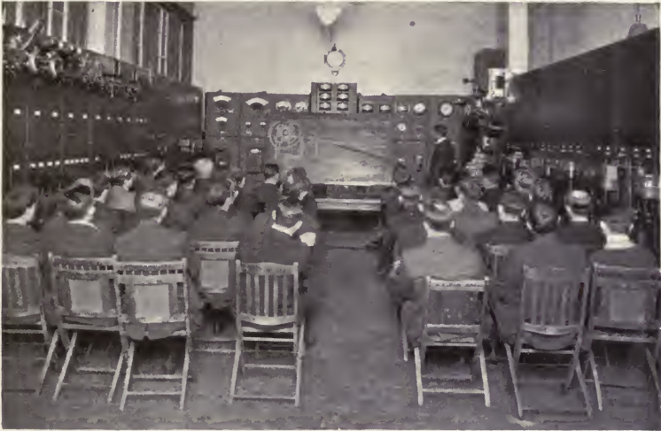
Fig. 87. SWITCHBOARD DEPARTMENT LECTURE
