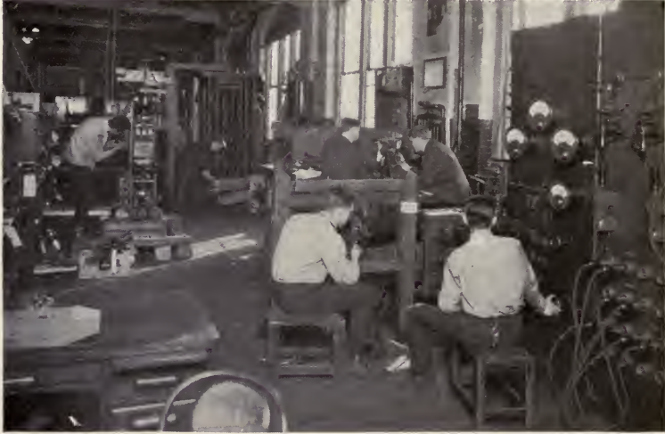
Fig. 88. TESTING SWITCHBOARD CIRCUIT BREAKERS AND RELAYS
