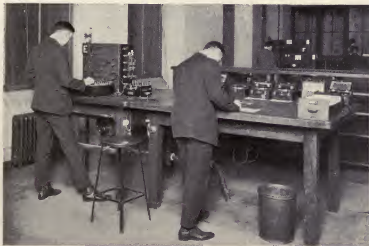
Fig. 81. CALIBRATING AMMETERS AND VOLTMETERS
