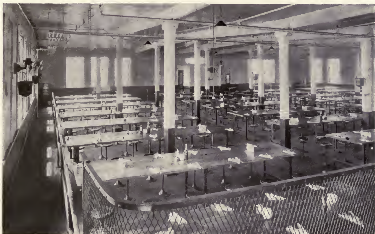
Fig. 63. FACTORY RESTAURANT, WEST LYNN WORKS
