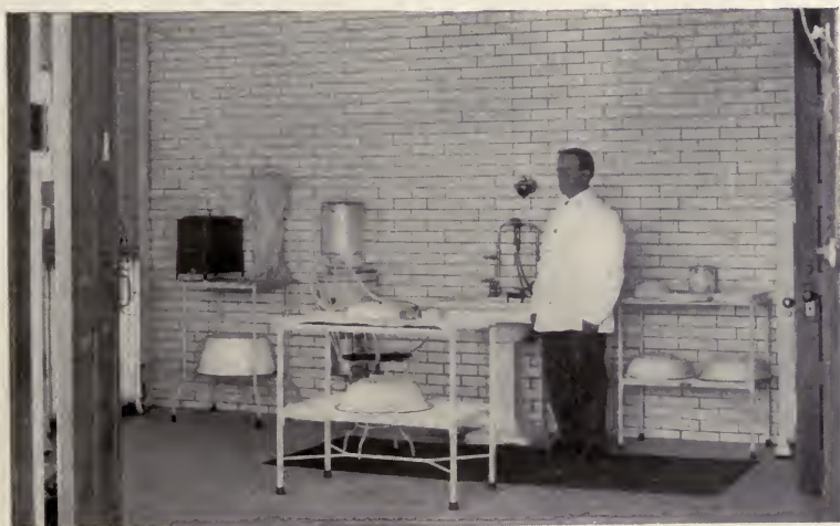
Figs. 32 and 33. THE PITTSFIELD WORKS HOSPITAL
