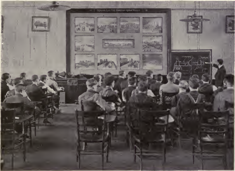
Fig. 65. INSTRUCTION IN MACHINE WORK AT LYNN WORKS
