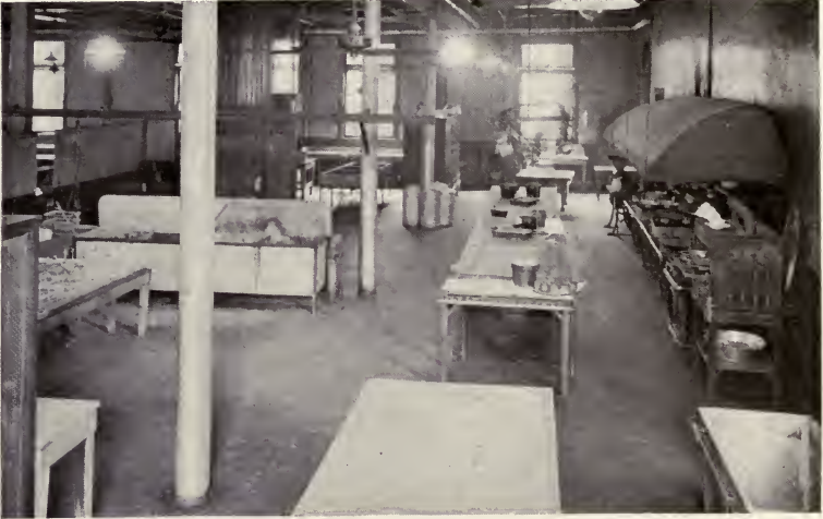
Fig. 53. KITCHEN IN SCHENECTADY WORKS RESTAURANT
