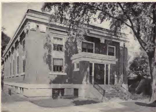
Fig. 4. EDISON HALL CONTAINS AN ASSEMBLY HALL, SEATING 400 PEOPLE; FOUR BOWLING ALLEYS, SHOWER BATHS, MOTION-PICTURE MACHINE, AND KITCHENETTE. THE MEETINGS OF THE A.I.E.E. AND OTHER ENGINEERING SOCIETIES ARE HELD HERE AND BY REMOVING THE PORTABLE CHAIRS A BEAUTIFUL BALLROOM FLOOR IS AVAILABLE FOR DANCING
