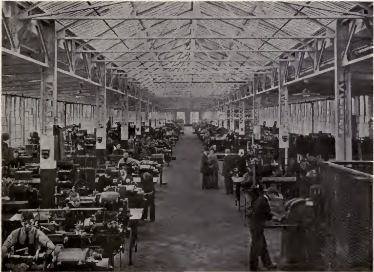
Fig. 73. TRAINING ROOM FOR MACHINIST APPRENTICES, LYNN WORKS
