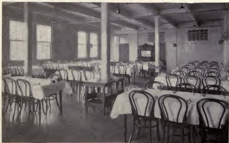
Fig. 58. FOREMEN'S DINING ROOM, WEST LYNN WORKS
