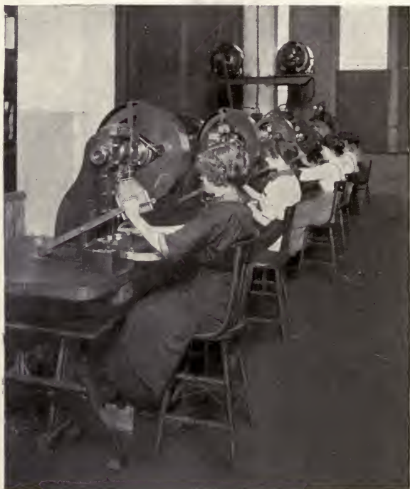
BATTERY OF PUNCH PRESSES EQUIPPED WITH "SIMPLICITY" GUARD IN OPERATION. PRESS CANNOT BE OPERATED WHILE GUARD IS UP
