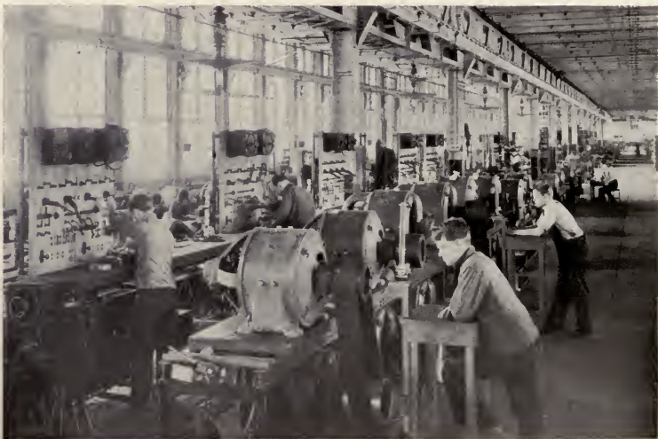
Fig. 83. COMMERCIAL TEST OF DIRECT-CURRENT MACHINES
