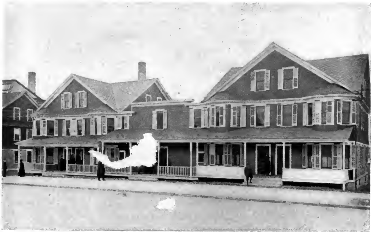
Fig. 52. PITTSFIELD WORKS RESTAURANT
