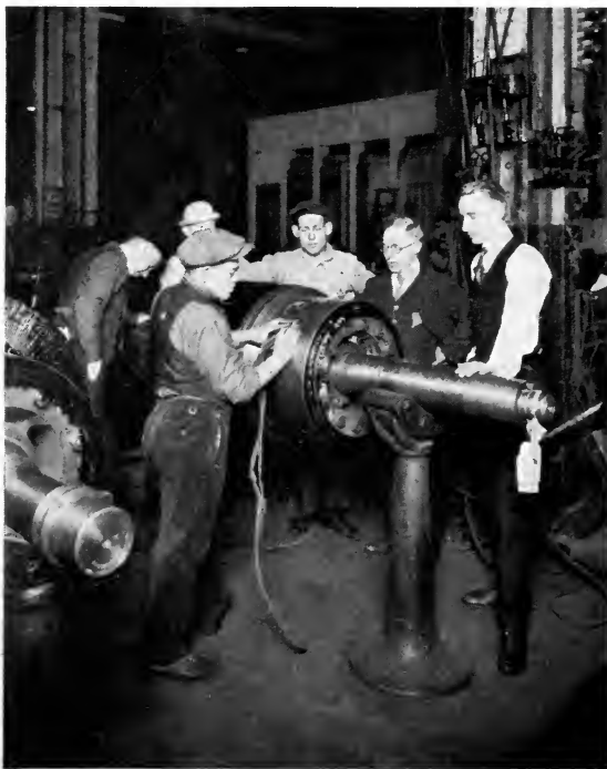
Fig. 85. LEARNING HOW TO TEST A MOTOR ARMATURE
