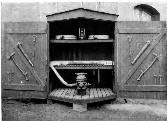
INTERIOR OF HOSE HOUSE, SHOWING FOUR-WAY HYDRANT, HOSE, AND OTHER EQUIPMENT
