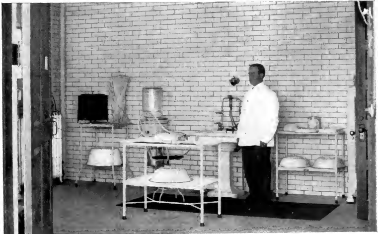
Figs. 32 and 33. THE PITTSFIELD WORKS HOSPITAL
