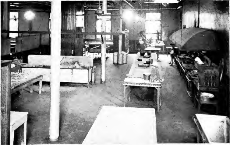
Fig. 53. KITCHEN IN SCHENECTADY WORKS RESTAURANT
