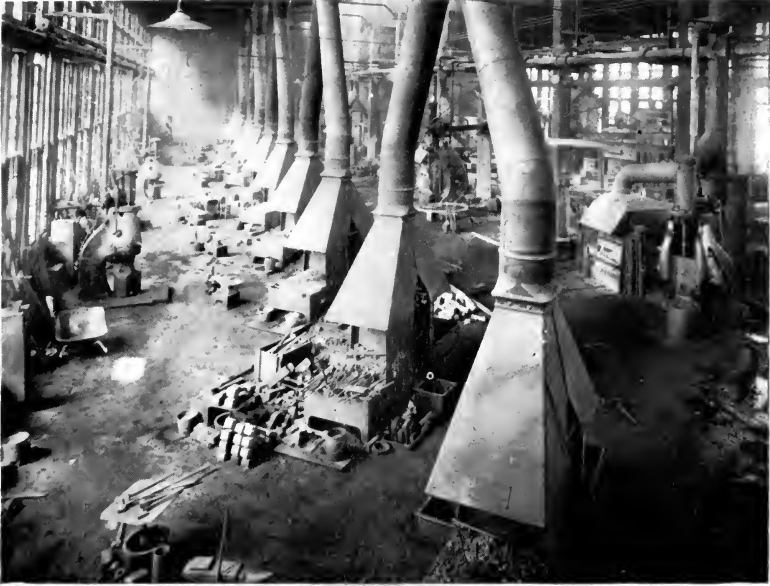
LIGHT AND VENTILATION IN BLACKSMITH SHOP
