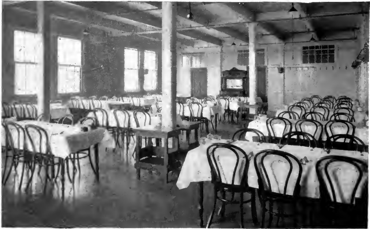
Fig. 58. FOREMEN'S DINING ROOM, WEST LYNN WORKS
