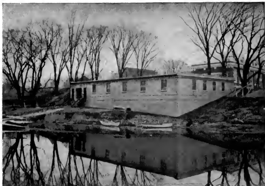
Fig. 7. THE CONCRETE BOATHOUSE ON THE BANKS OF THE MOHAWK RIVER IN THE REAR OF EDISON CLUB AND HALL. A DOUBLE TRACK IS PROVIDED FOR RUNNING THE 200 CANOES IN AND OUT OF THE FIREPROOF BOATHOUSE
