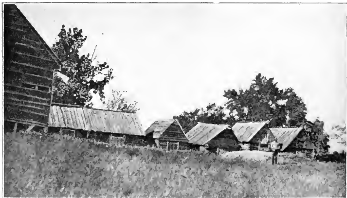
Log Cabin, Corn Houses and Barns, on Wakefield Estate, the Birthplace of George Washington.
