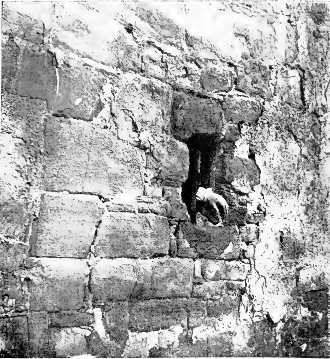
OLD WALL OF BALHOUSIE CASTLE, PERTH Used by Millais in his background of “James’ Love”
