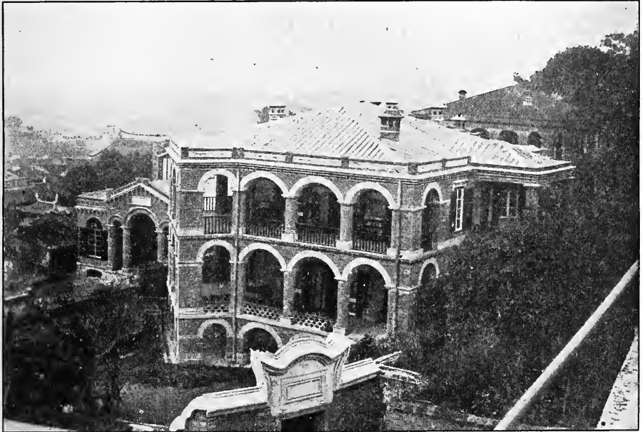
OPERATING PAVILION, DR. KINNEAR'S HOSPITAL, FOOCHOW CITY
