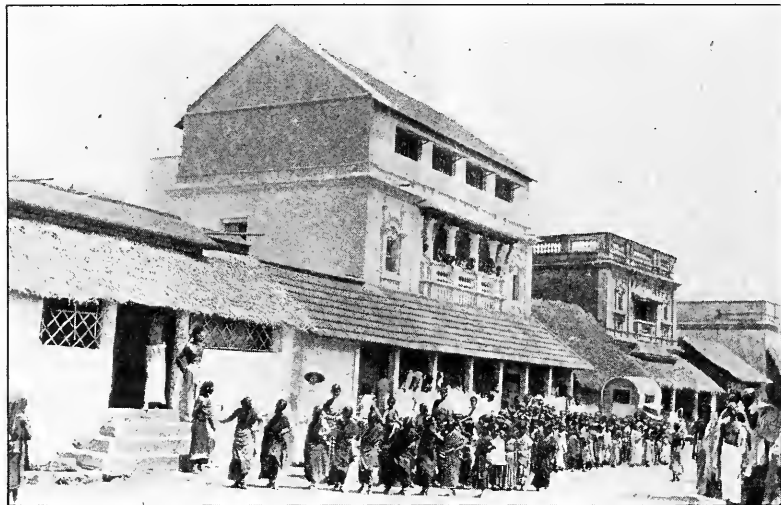
The New Kindergarten Addition in Aruppukottai
