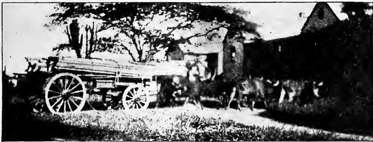
Hauling Timber for Industrial Building Inanda Seminary, South Africa. Golden Anniversary Gift
