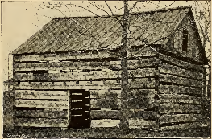
FIRST COURT-HOUSE AT DECATUR, ILLINOIS.
