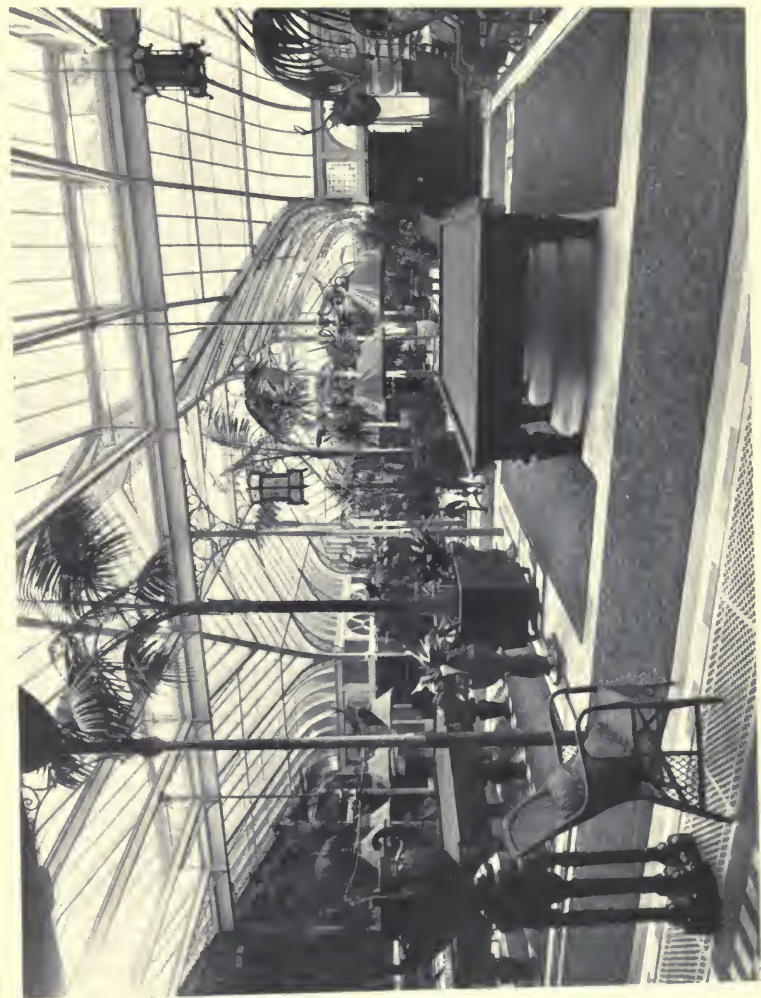
THE BILLIARD ROOM AND CONSERVATORY, LITTLETON PARK
