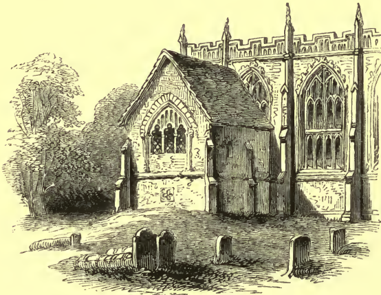
Exterior of the Charnel house, Stratford.
