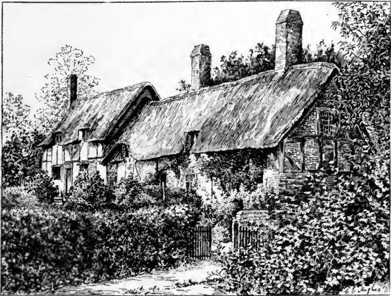
ANNE HATHAWAY'S COTTAGE AT SHOTTERY
