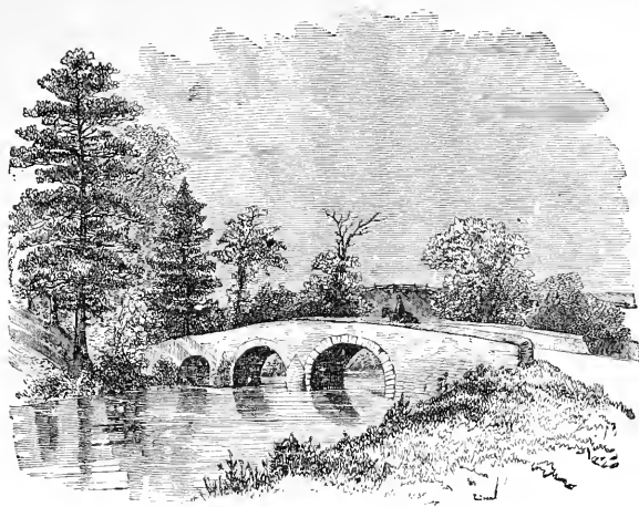
The Stone Bridge at Antietam.
