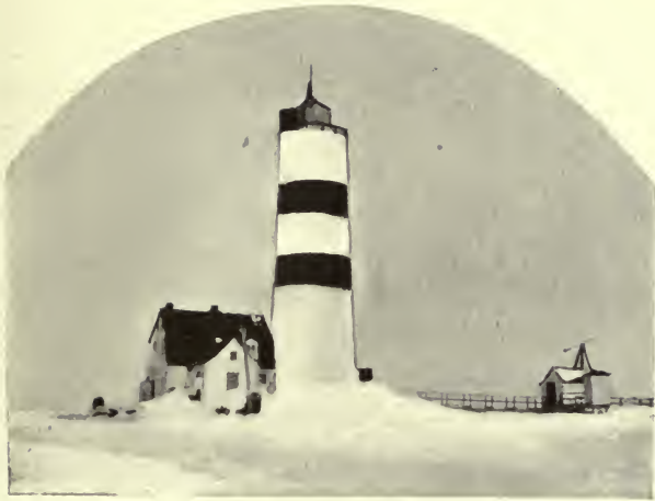
Pointe des Monts Light-House.
