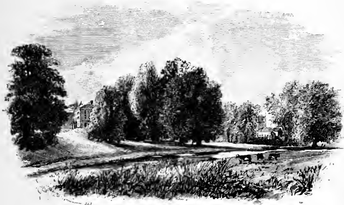
NETHER AVON HOUSE AND CHURCH.
