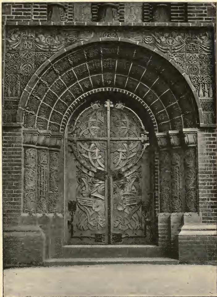
MORTUARY CHAPEL: PORCH AND DOOR.
