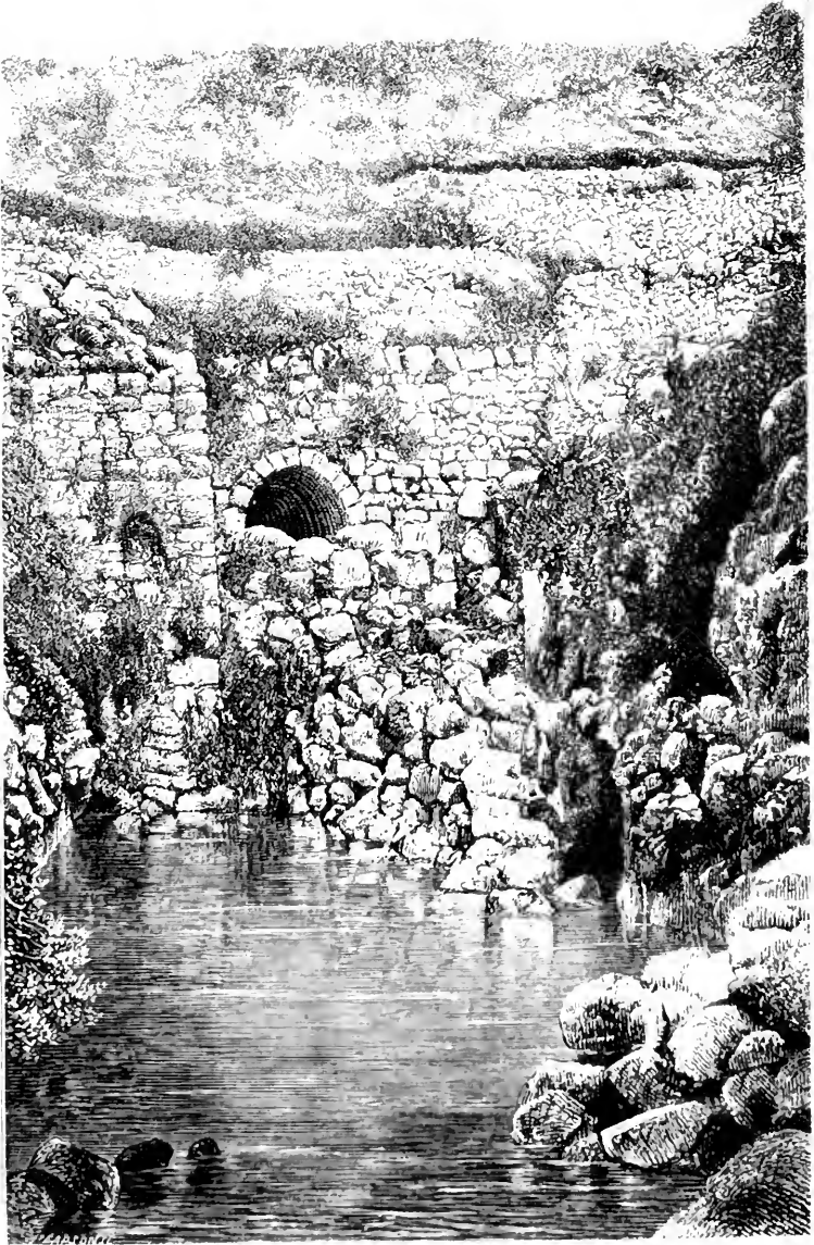
FOOT OF DAM
