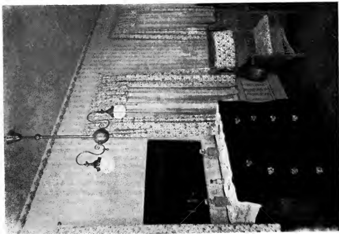
With the inverted mantle the major part of the light is downward, illuminating the features before the mirror.
