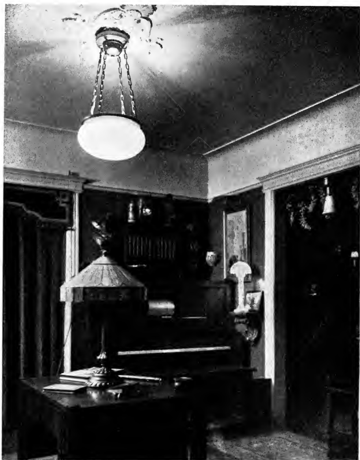
The objection to the opaque bodies often used in indirect lighting is overcome here. This is an indirect unit with a small additional light used simply to illuminate the art glass bowl.
