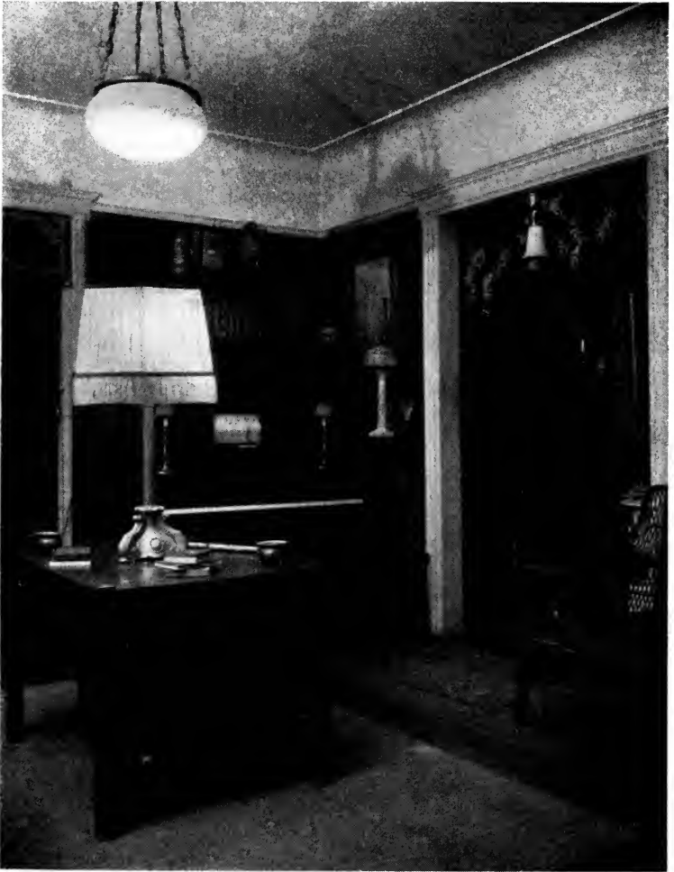
Indirect lighting is applicable to portable lamps. The powerful reflector throws the light upward to the ceiling whence it is diffused. Here the light is directed against the glass bowl which is used as a secondary source of distribution.
