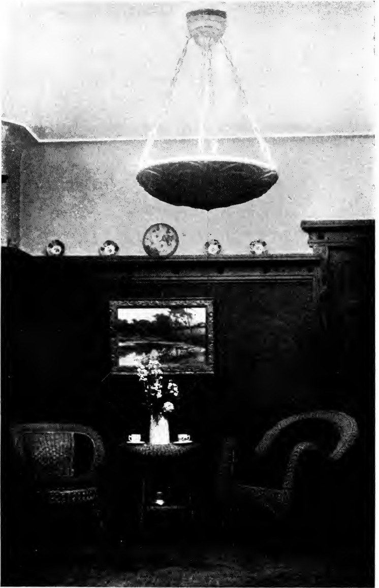
A corner of a room where standard indirect equipment is used. The reflectors throw the light upon the ceiling from whence it is diffused evenly about the whole room.
