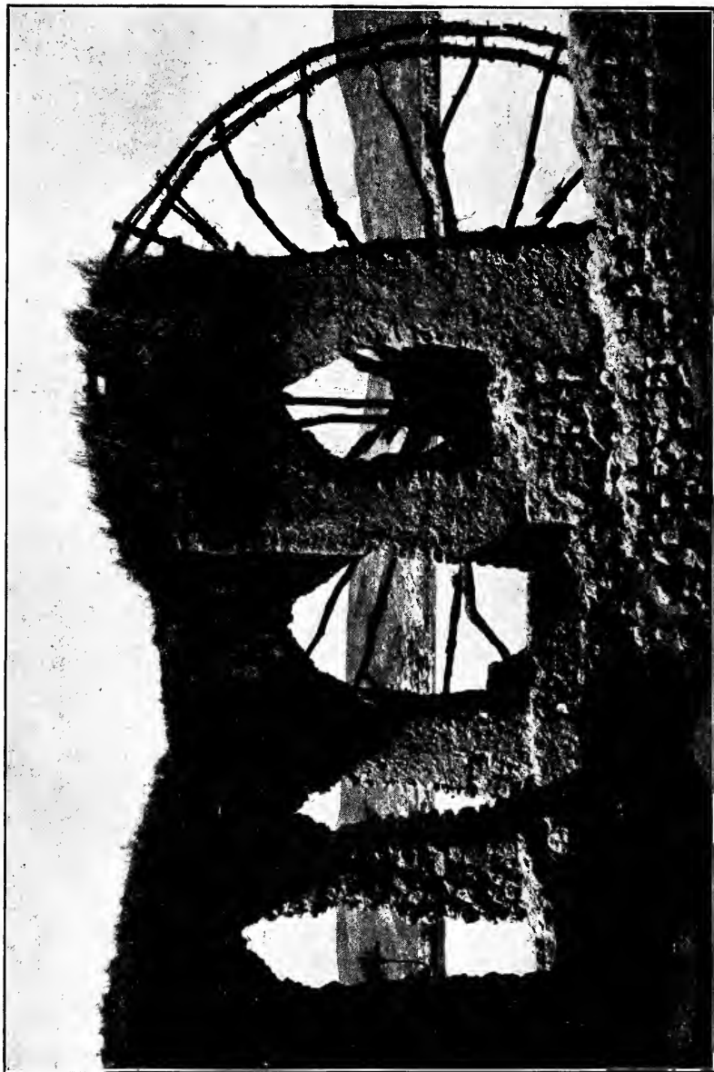
Modern water wheel or saqiya in Babylonia. The river is dammed up and the water made to pass the wheel to which, when in use, paddles were attached and bottles were attached to lift the water to the aqueduct.
