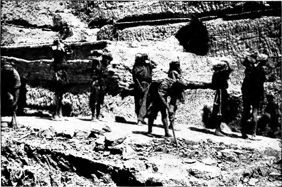
Workman removing the pavement containing bricks with the titles of Sargou and Narâm-Sin.
