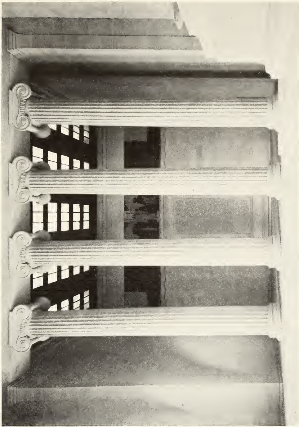
The south wall, through Ionic columns
