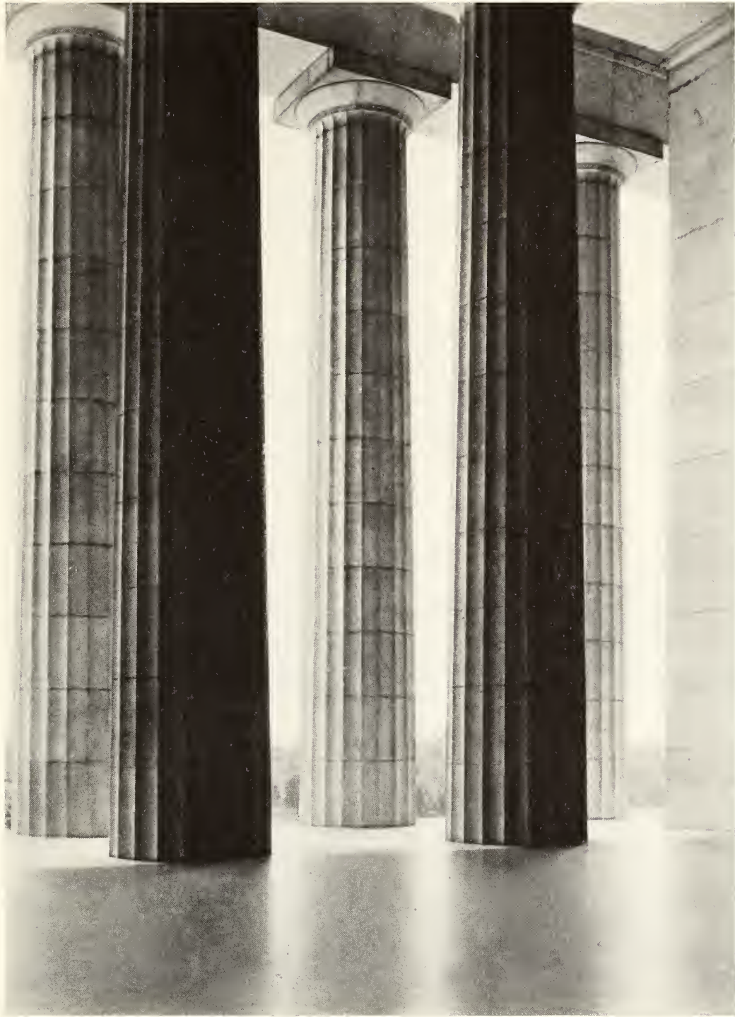
The portal, looking southeast
