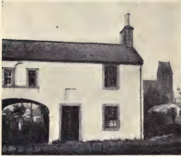
ARCH HOUSE, ECCLEFECHAN
