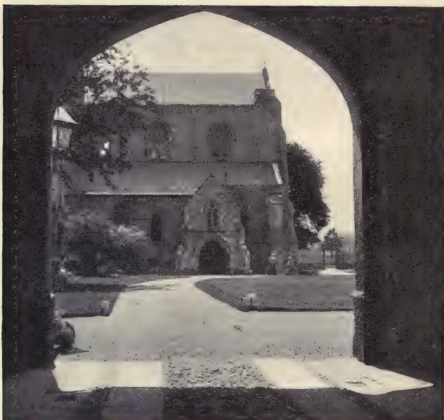
THE ENTRANCE TO ST. CROSS
