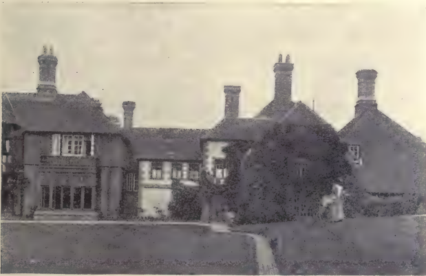
GILBERT WHITE'S HOUSE FROM THE REAR
