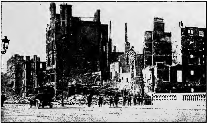
RUINED BUILDINGS IN SACKVILLE STREET, DUBLIN, DUE TO THE INSURRECTION
