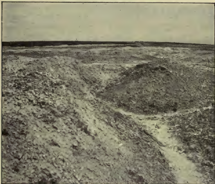
A GERMAN TRENCH ON THE SOMME AFTER IT HAD BEEN BOMBARDED
