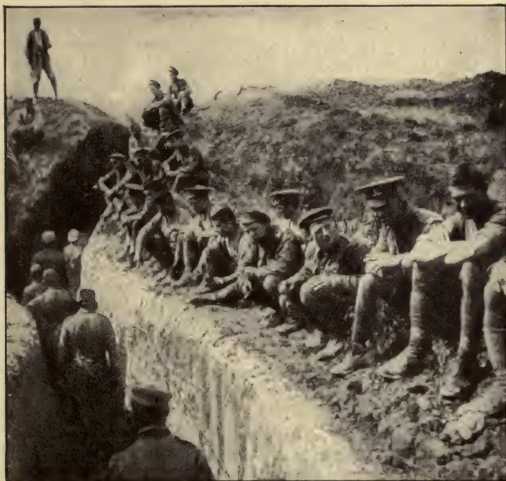
IN A WESTERN TRENCH
