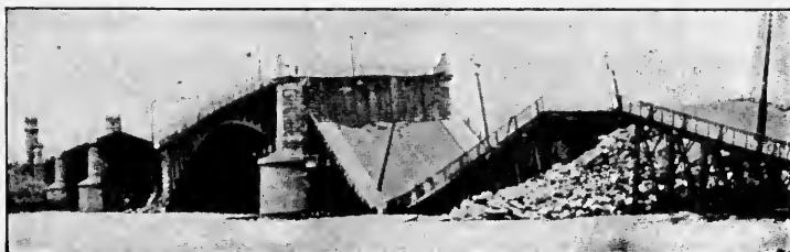
WARSAW BRIDGE WRECKED BY THE RUSSIANS BEFORE THEY EVACUATED THE CITY
