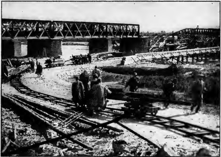
REPAIRING A DAMAGED RAILWAY-BRIDGE ON THE DUNAJEC RIVER
