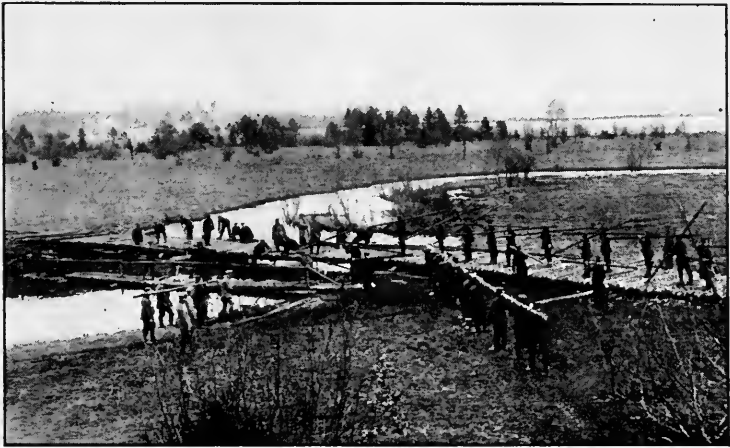
GERMANS BUILDING A BRIDGE ON THE RUSSIAN FRONTIER
