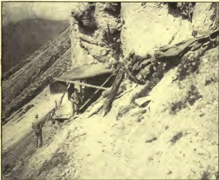
AN AUSTRIAN SHELTER IN THE ALPS
