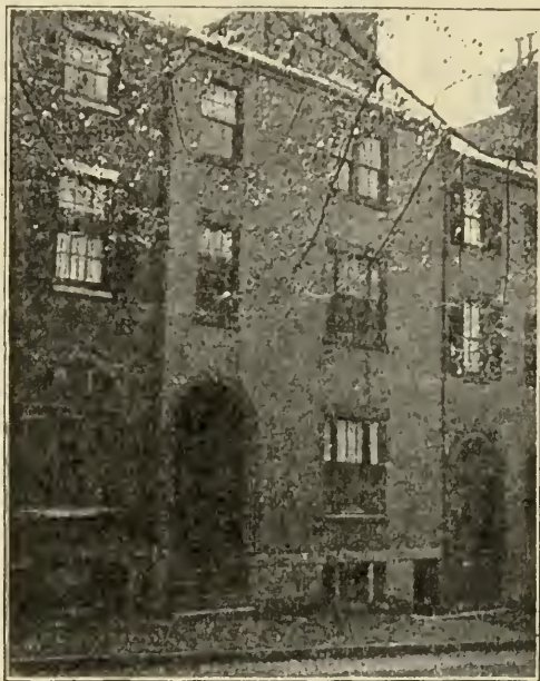
HOME OF FRANCIS PARKMAN CHESTNUT STREET
