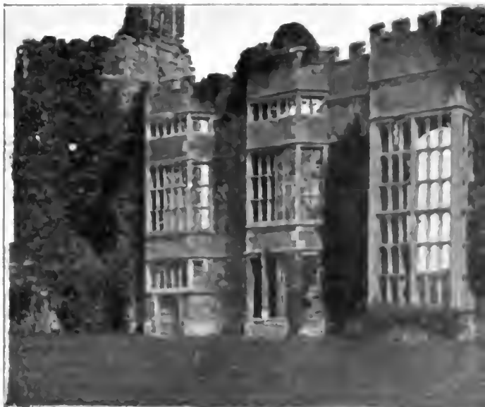
COWDRAY HOUSE, SUSSEX. PART OF COURT. Small Gothic Window (on the right), Tudor Bay Window next to it (to the East) on the left.
