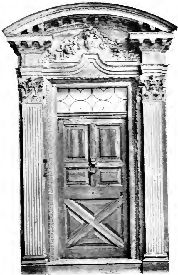
FIG. 1. DOORWAY EARLY EIGHTEENTH CENTURY
