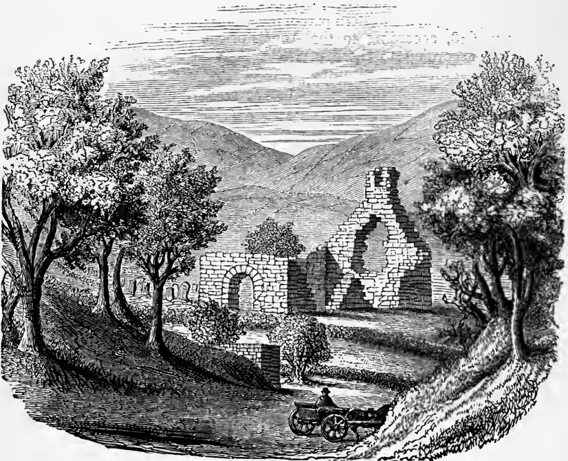
Old Church at Dysart Gallen, Queen's County.
