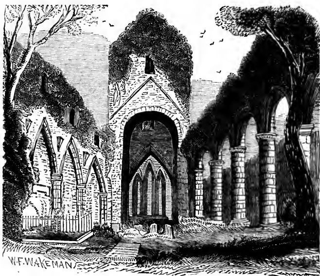
Interior of Boyle Abbey, County of Roscommon.
