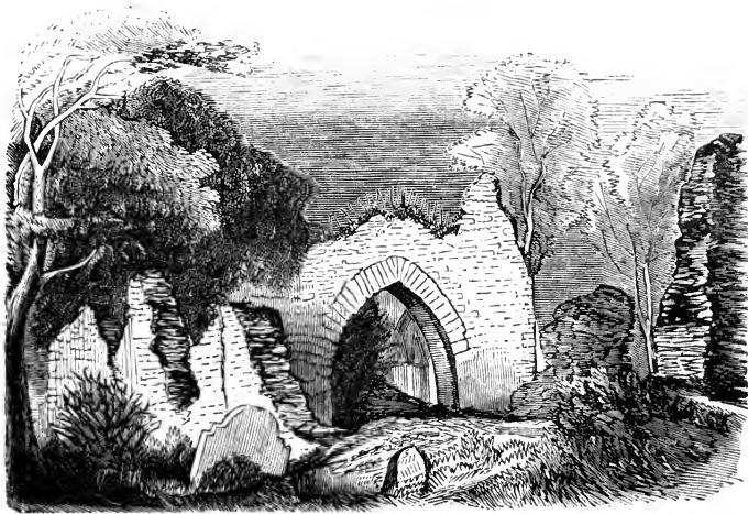
Coolbanagher Old Church, Queen's County
