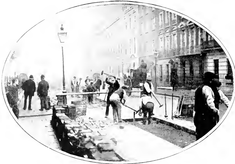
LAYING ELECTRIC CABLES (WIGMORE STREET).
