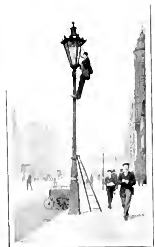
SUPPLYING ARC LAMP WITH CARBON.
