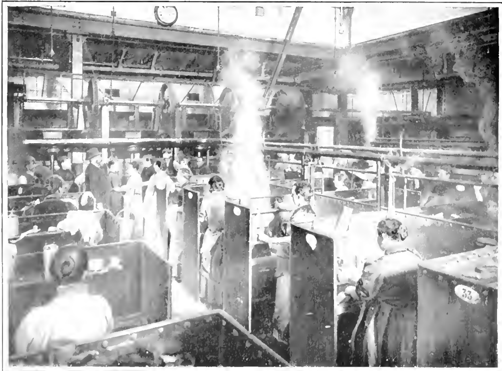
N. A. P. U. B. WASH-HOUSE (MARLBORNE ROAD) : WASHING.
