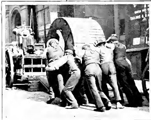
I. WIRE REPAIRERS AT WORK. II. A REEL OF WIRE.
