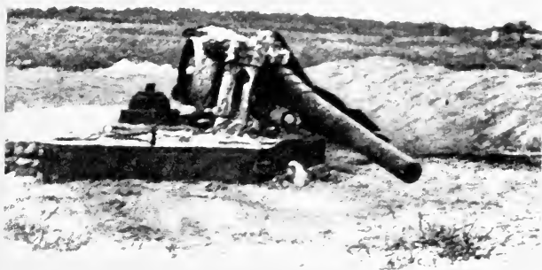
WEST BATTERY, CAUVÉ, AFTER DESTRUCTION
