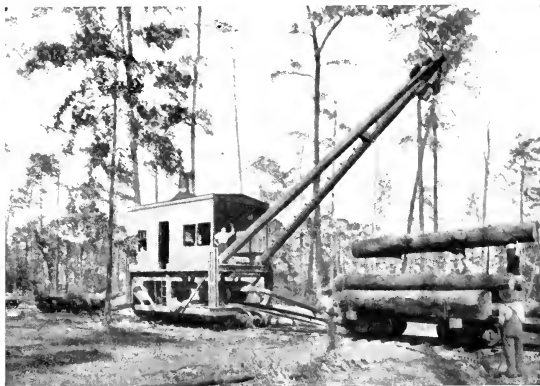
FIG. 94. — A Decker Log Loader.
