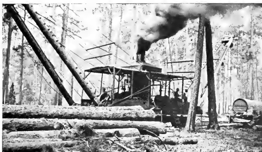
FIG. 57. — A Portable Snaking Machine operating in a Texas Longleaf Pine Forest.
