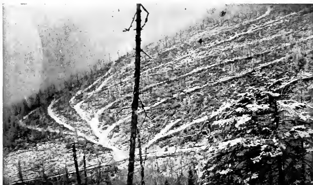
FIG. 37. — Yarding-sled Trails leading down to a Skidway on a Two-sled Road. Maine.
