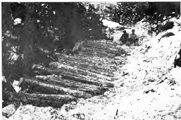
FIG. 39. — A Two-sled Road, showing the Method of building up the Grade on Side Slopes.
