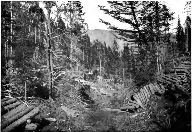
FIG. 26. — Skidways along a Two-sled Road. Montana.
