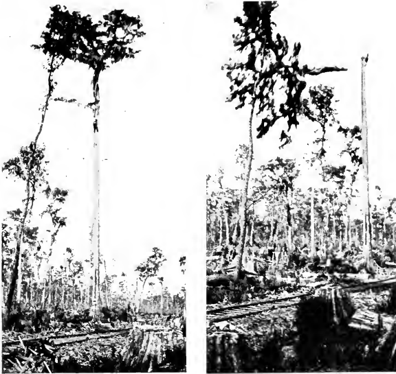
FIG. 55. — Cutting the Top from a Head Spar on which is placed the Main Cable Rigging for a Cableway Skidder. Cypress Forest, Louisiana.
