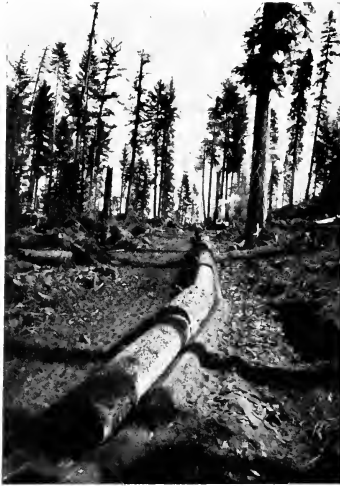
FIG. 67.—A Fore-and-aft or Pole Road used with a Road Engine. Pacific Coast.
