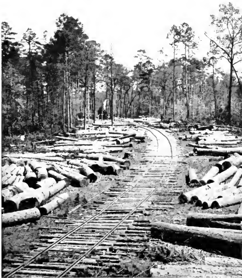
FIG. 80. — A Spur Logging Railroad corduroyed with Poles. Arkansas.
