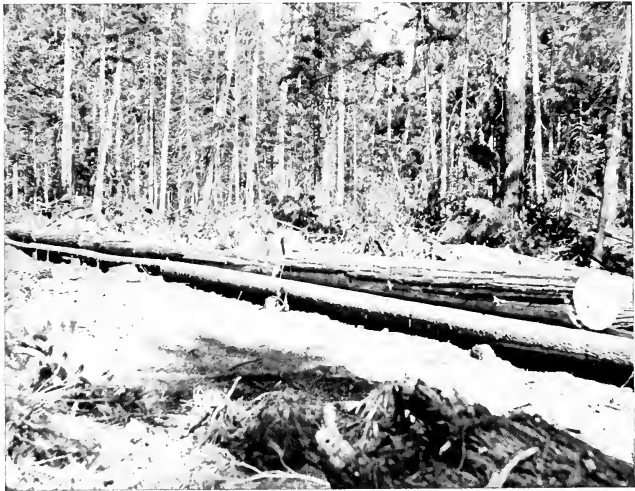
FIG. 69. — A Turn of Logs ready to move along a Trailing Slide.
