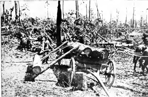
FIG. 50. — Loading a Log Wagon by means of the Cross-haul. Missouri.
