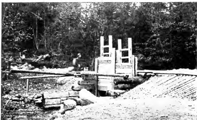
FIG. 100. — The Upstream Face of a Small Rafter Dam, showing a Common Form of Lift-Gate.
