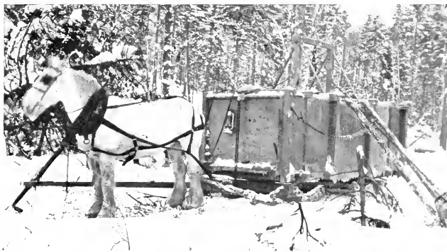
FIG. 41. — A Sprinkler being filled with Water from a Brook. Maine.
