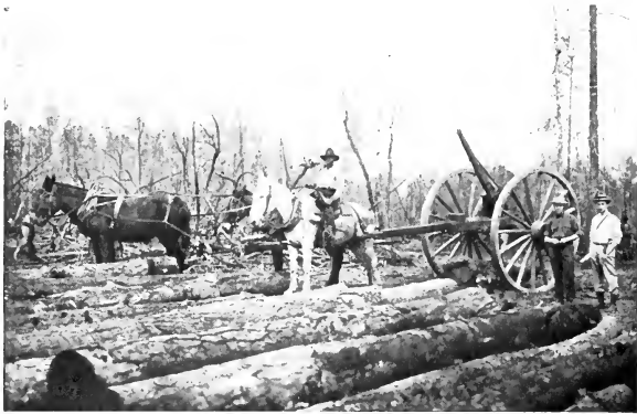
FIG. 47. — A Slip Tongue Cart in a Southern Yellow Pine Forest. Lever arm is elevated so that the grabs can be removed from the logs. Texas.
