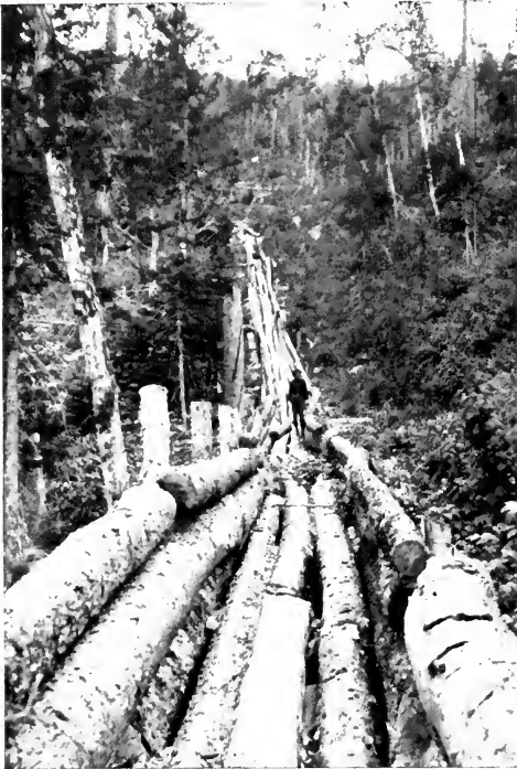
FIG. 68. — A Timber Chute. New Hampshire.
