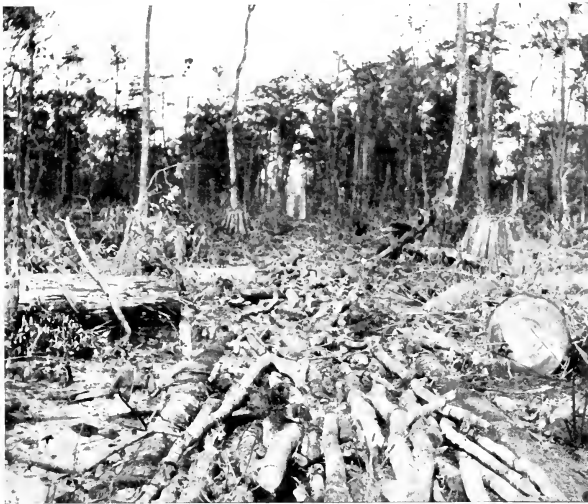
FIG. 79. — The Foundation for a Dunnage Road. Louisiana.
